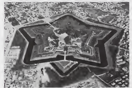
Goryokaku Park, Western-style fort constructed in the mid-19th century in Hakodate, Japan
